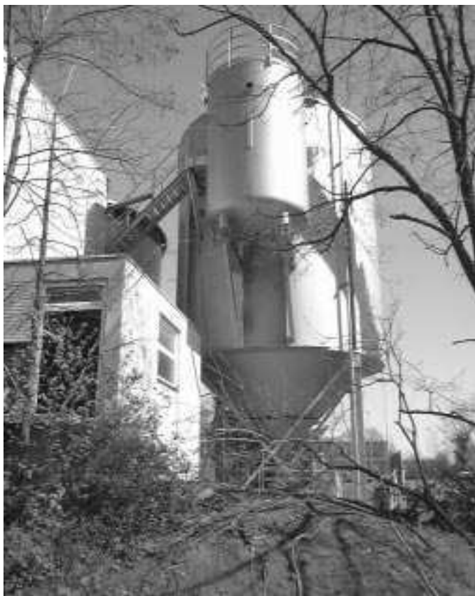
Fig. 9.6 Lime softening plant (Source: EUWA).
