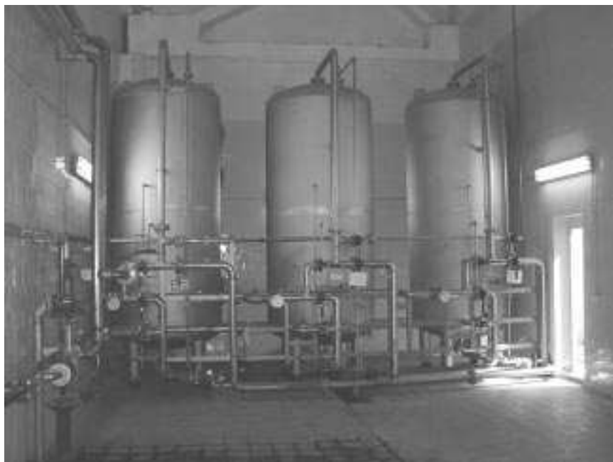
Fig. 9.4 Activated carbon filter plant (Source: EUWA).
